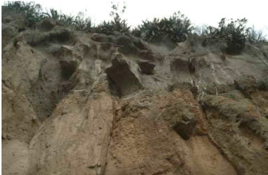
Fig. 6 – The Rock of Orvieto before the stabilization works. You can note the columnar fracturing affecting the tuffaceous mass (photo by P. Marconi).
